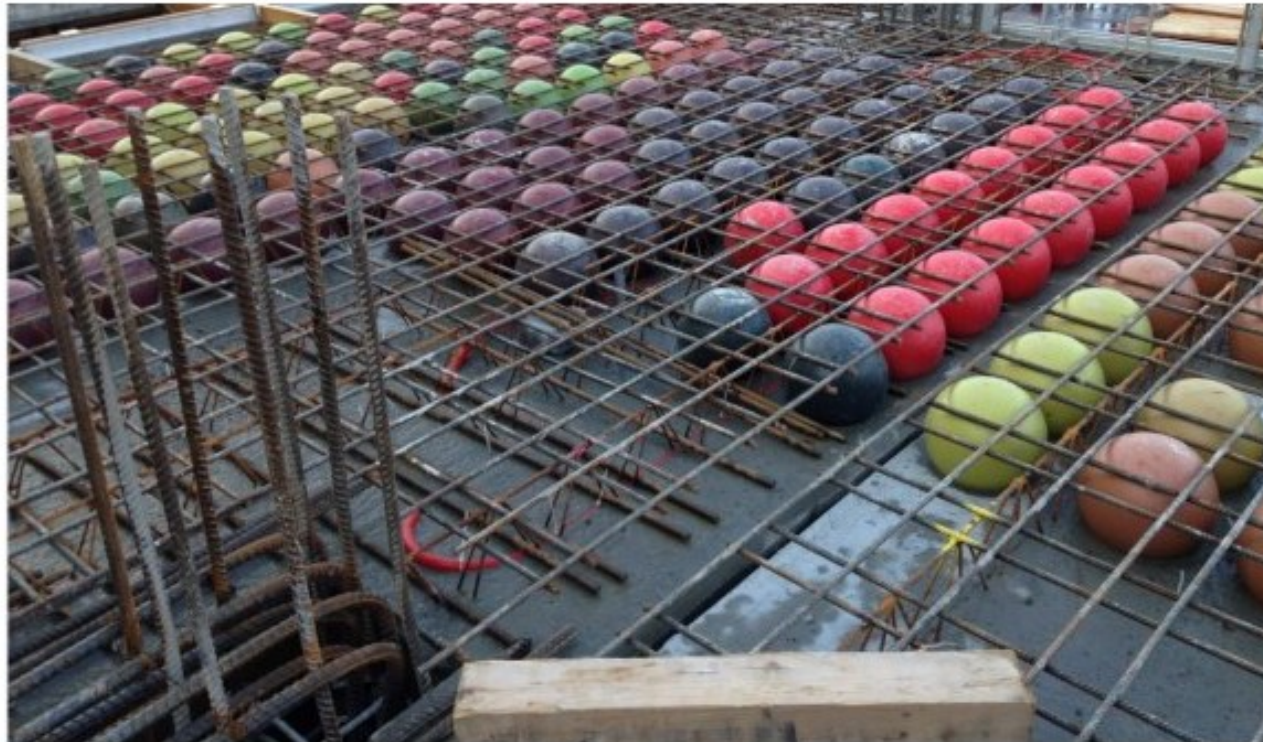
Bubbledeck panels placed on site. Bubbles have been omitted around the zone of influence of columns, where punching shear forces are high, and additional reinforcing is required. (photo courtesy Bubbledeck North America)
